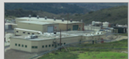
Main Control Facility
