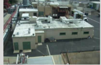
HEPTS Control Center
