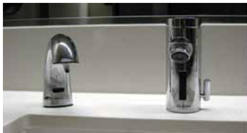
Newly upgraded restrooms in the El Segundo Continental Building include features that save water and energy as well as reduce solid waste. The sink (above) features a faucet with a low-flow aerator to conserve water and an automatic soap dispenser to reduce waste.
